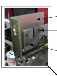
Connecting Bracket – Align 1<sup>st</sup> to existing holes in breaker frame.
